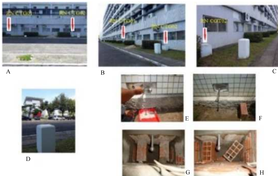
Fig. 1: TGC Level References: A. TGC school building and front facade; B. Front view to the right of the RN CTG01 and RN CTG02; C. Front view to the left of RN CTG02; D. Building LITPEG/UFPE built and view of RN CTG 02 to the building; E. a H. Materialization of the RN CTG01 and RN CTG02
