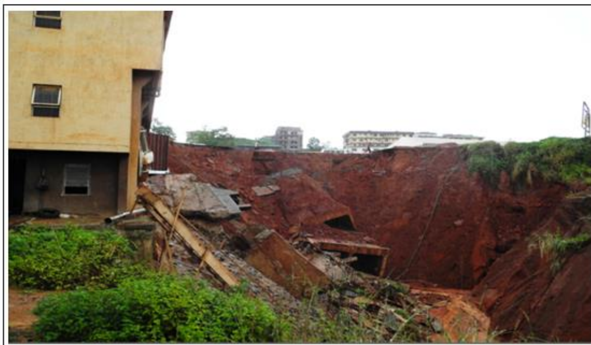
Fig. 1: Gully erosion in Onitsha southeast Nigeria (Abdulfatai et al. , 2014)
