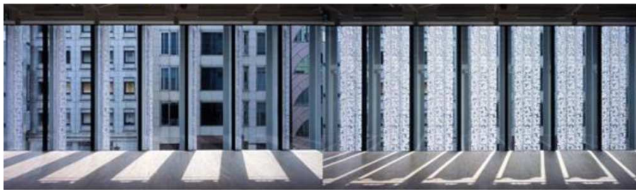
Fig. 9: Pola Ginza Building Facade, Tokyo, Japan (adapted from (Marysse, 2016))
